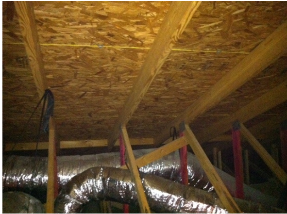
Attic with no radiant barrier protection
