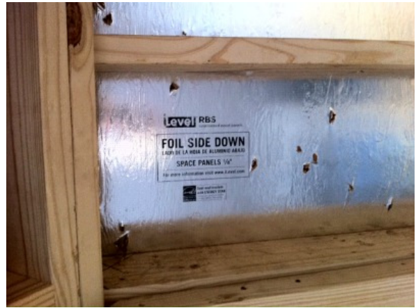
OSB decking with radiant barrier
