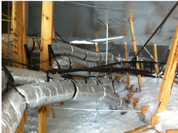
Rafter-applied sheet radiant barrier
